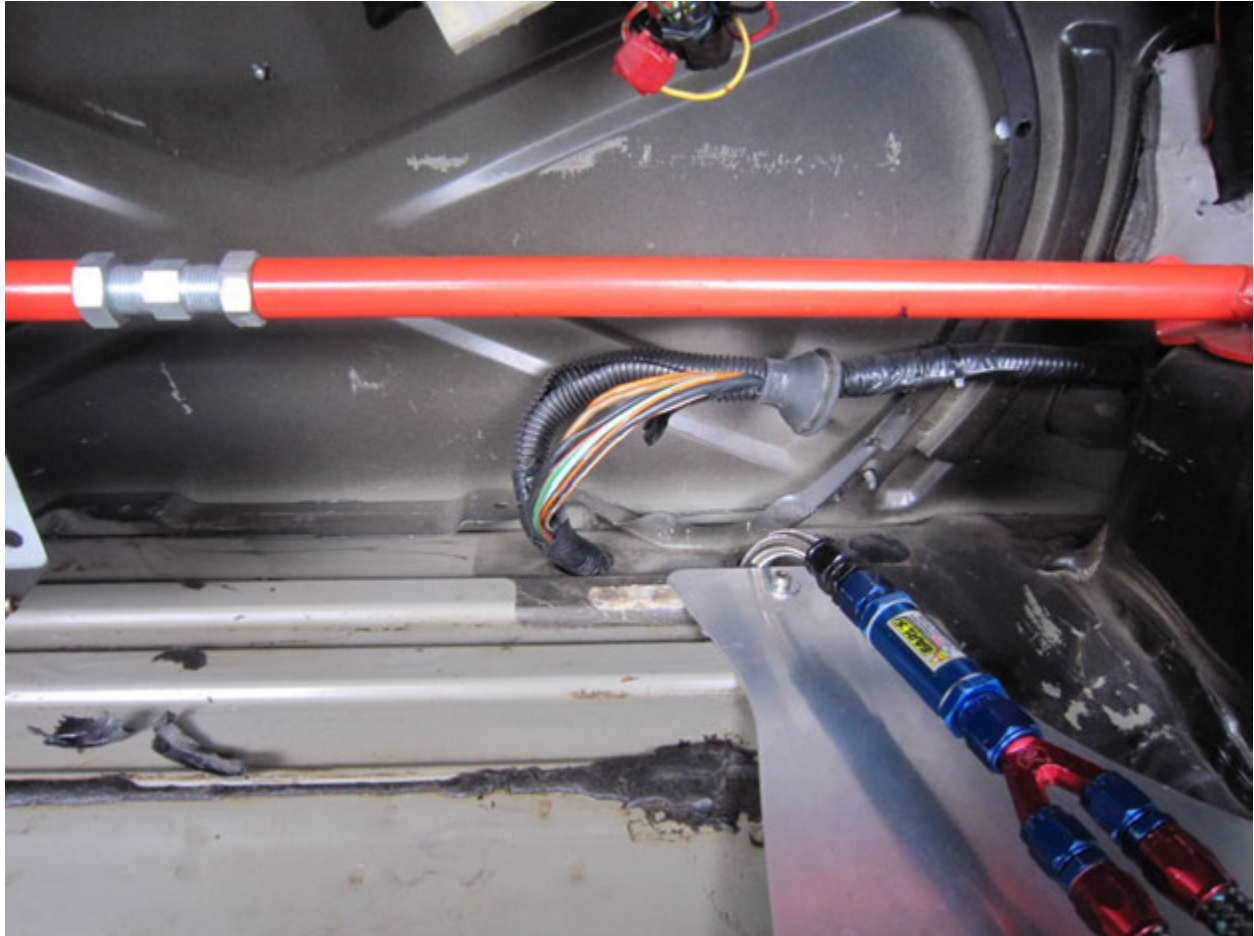
Shows tracing the wires back to the loom at the front of the boot space.
